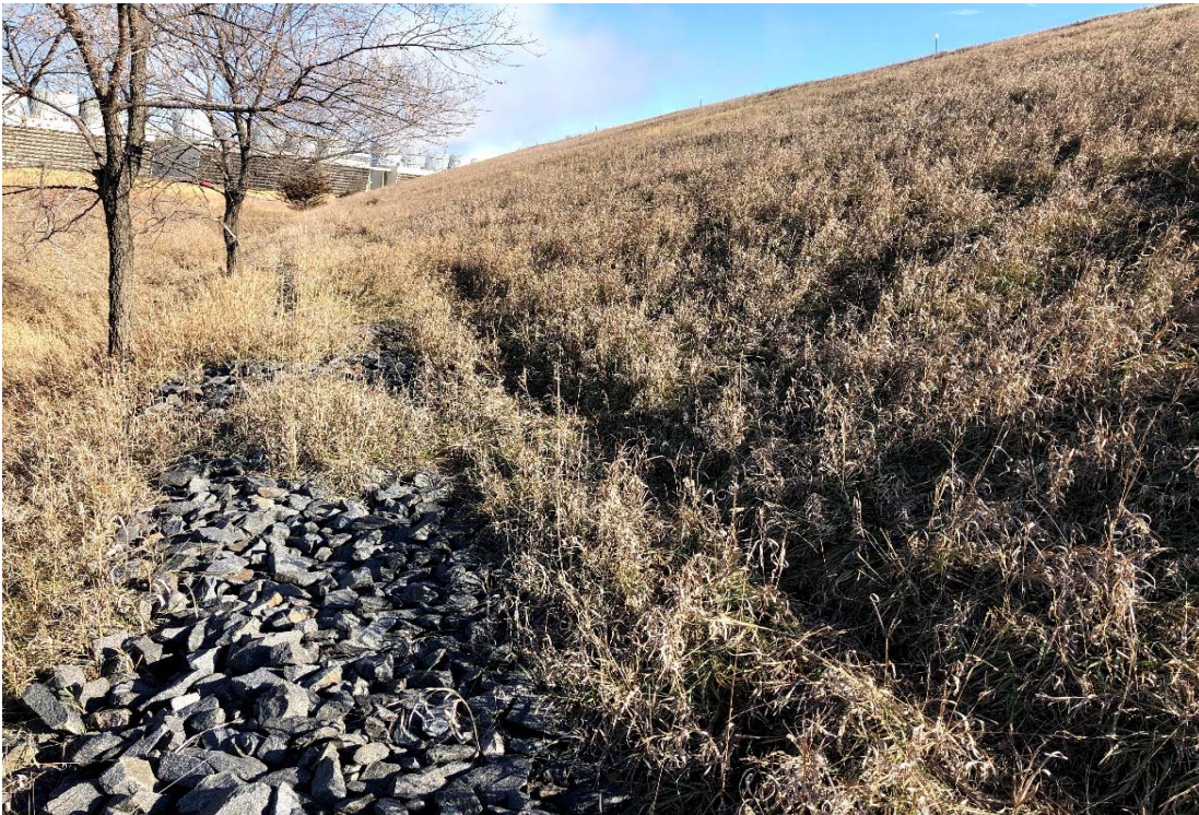
Photo 10 Mid-slope exterior of northwest embankment with toe drain, looking northeast. 11/19/2020
