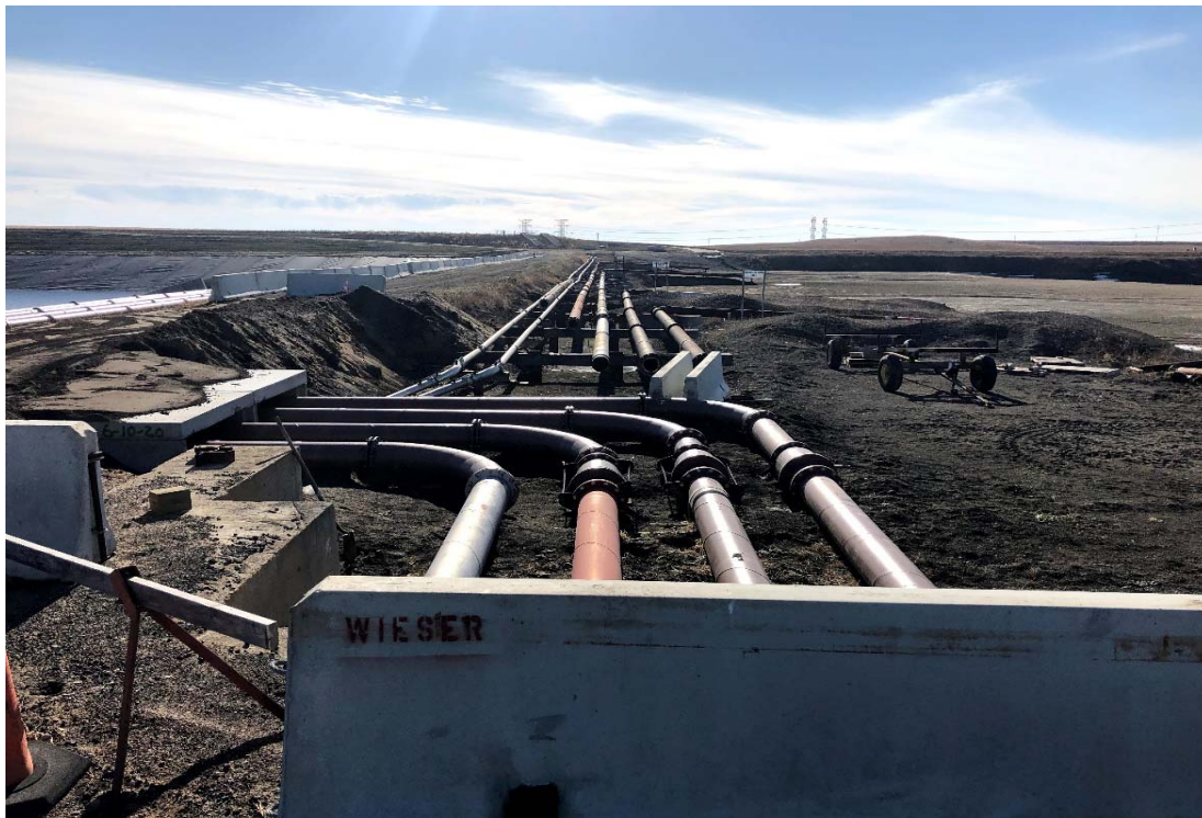
Photo 2 Interior of east embankment, looking south. Bottom ash pipe routed to new pond (Bottom Ash Pond 2). 11/19/2020
